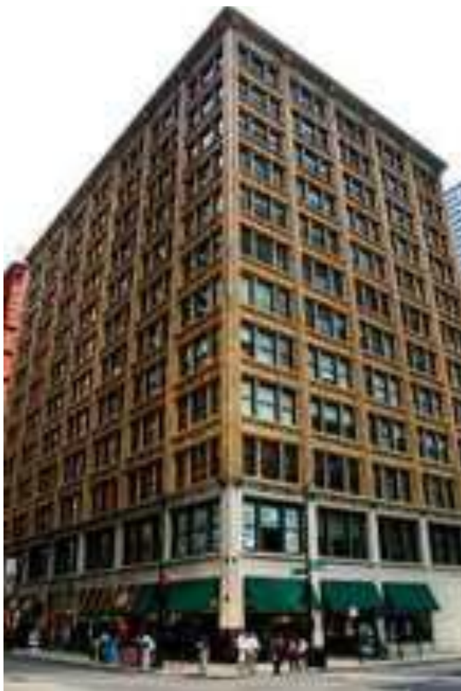
Foto: Brooks Building , Chicago.
